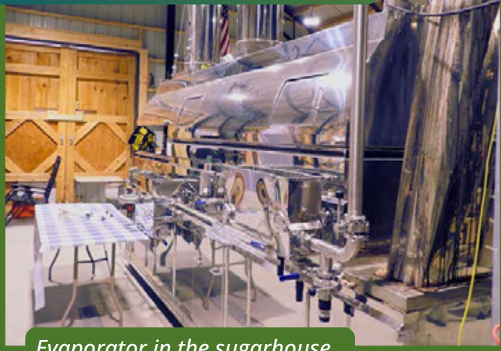
Evaporator in the sugarhouse.
