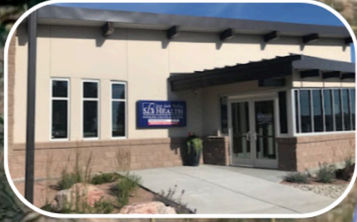
San Luis Valley Health Conejos County Hospital
