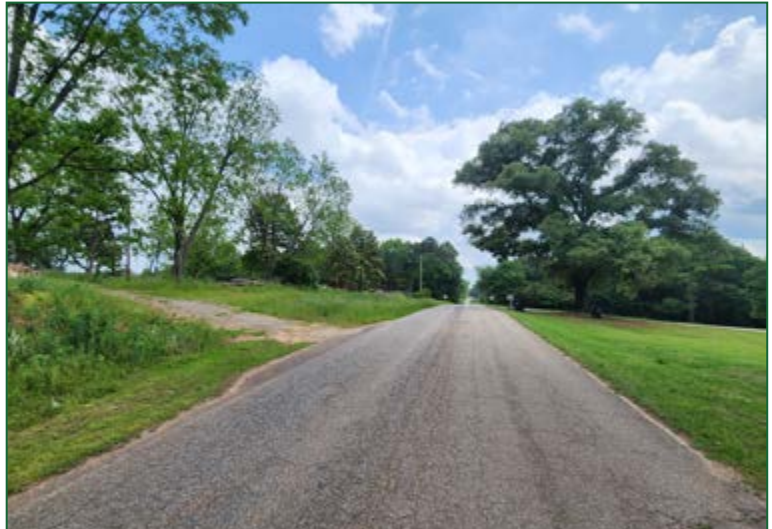
Entrance of the tract facing south along County Road 57.
